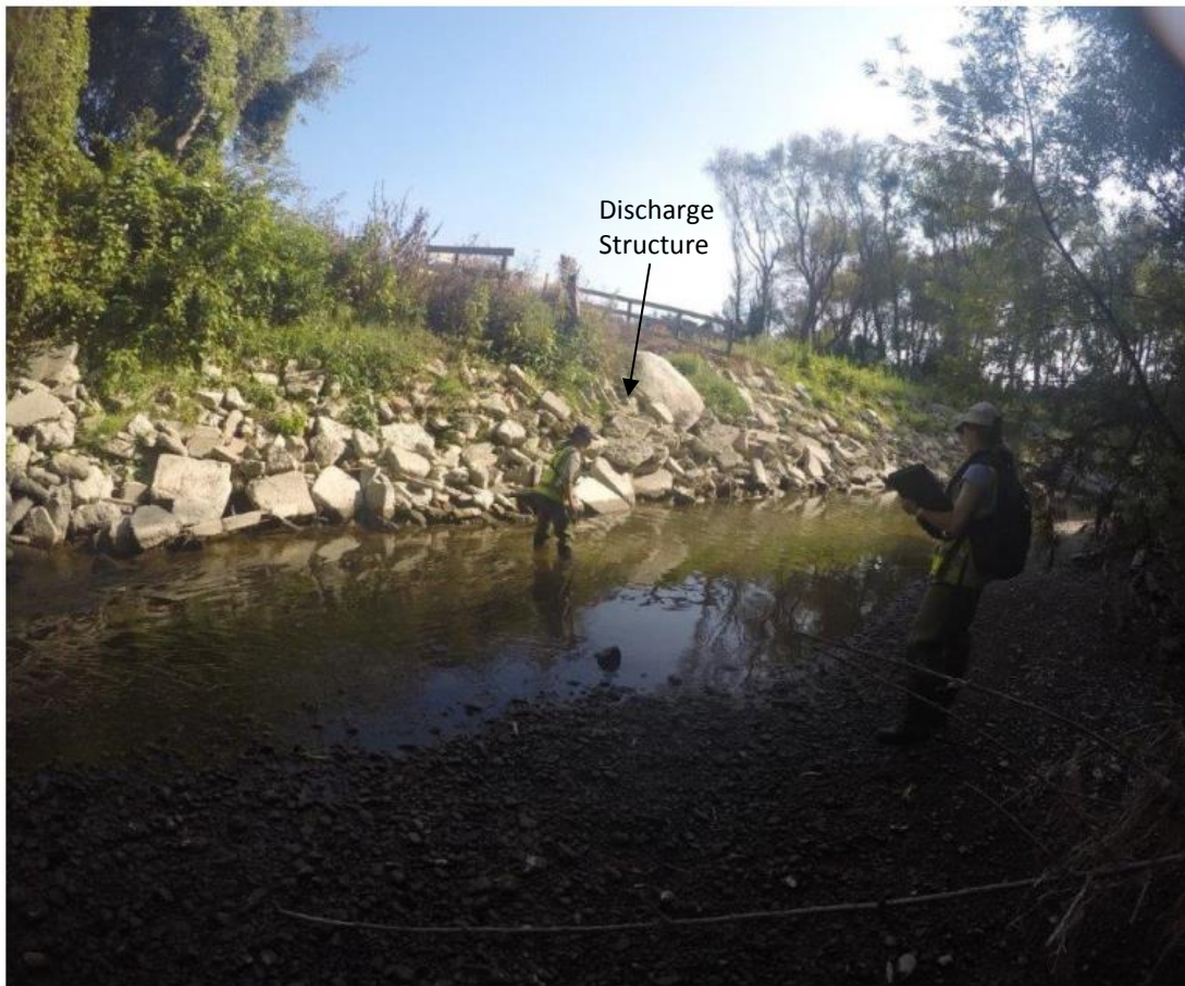
Figure 3.1: Discharge Site (Note: Wastewater flows through the sub-surface of the rock structure)
